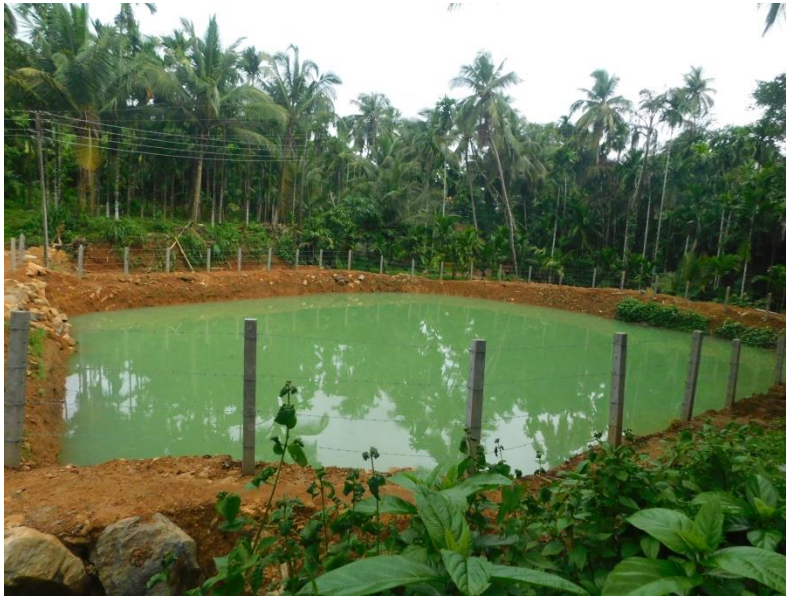
Figure 1 Mulia farm pond renovation completed on 28-6-2020
